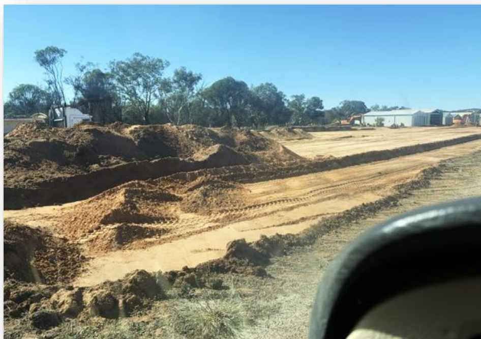
Earthworks Northam Aero Club 12 May 2026
